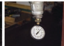
Pressure is relieved, and pipeline repairs can be made.
