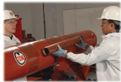
Wrap carbon fabric on pipeline.
