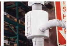
Work is complete and the ice plug is thawed.
