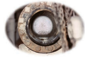
The Ice Plug is created in the pipe, forming a seal.
