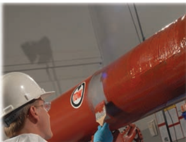
Apply epoxy to pipeline.
