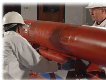
Wrap barrier fabric on pipeline.
